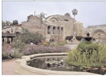
Built in 1779, the "Serra Chapel" at Mission San Juan Capistrano is the oldest church building in California.
